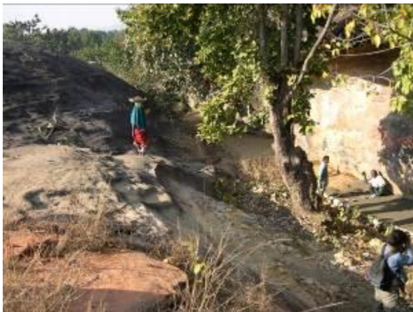
Breaking stone steps and cementing the floor of Isco rock-art shelter
