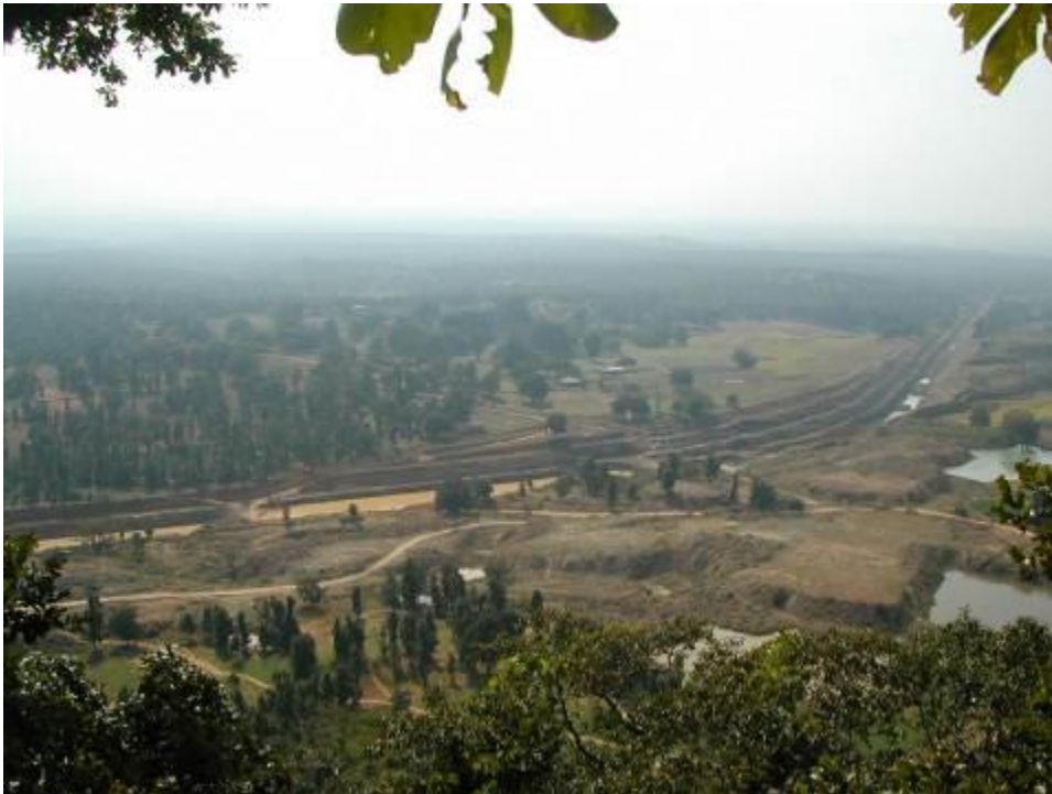
View of the railway line being built through archaeological site below the rock-art site
