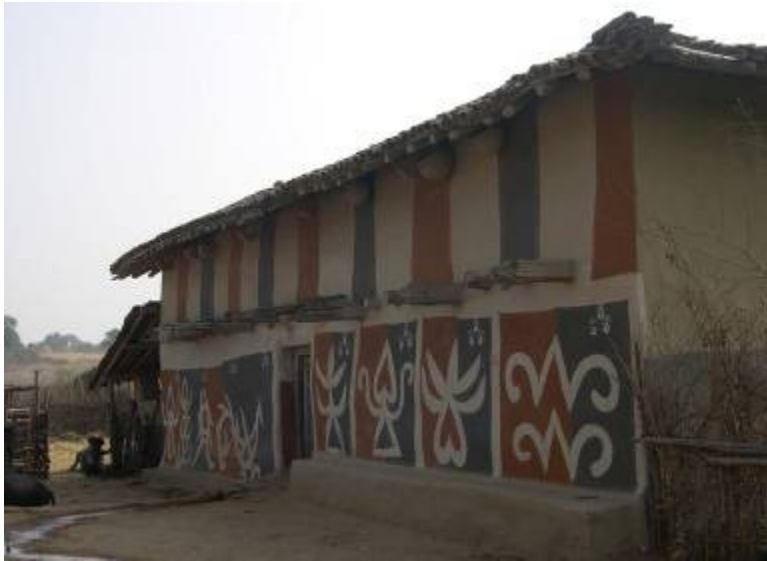
Kurmi Sohrai glyptic wall painting (Bhelwara)
